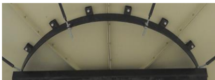
Figure #7 Back Brace To Clip
